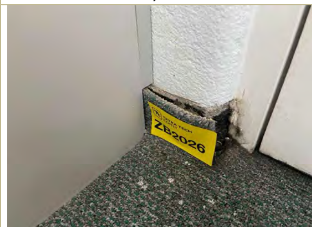
Item Number 6: Internal, L1, Beneath carpet, South elevation, Black tile, Vinyl Floor Tile - Chrysotile
