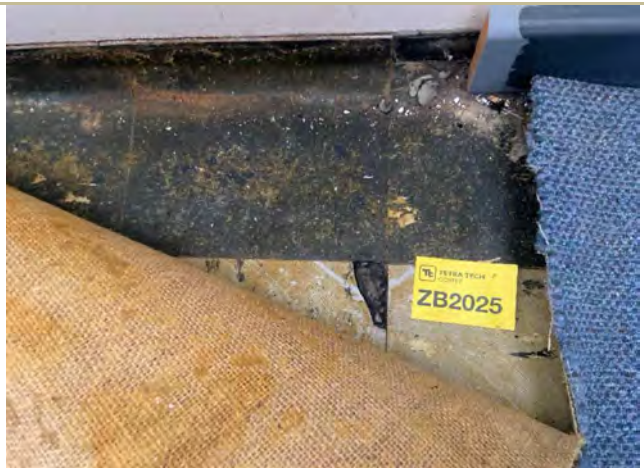
Item Number 4.1: Internal, L1, Beneath carpet, South elevation, light blue tile, Vinyl Floor Tile and glue - Chrysotile
