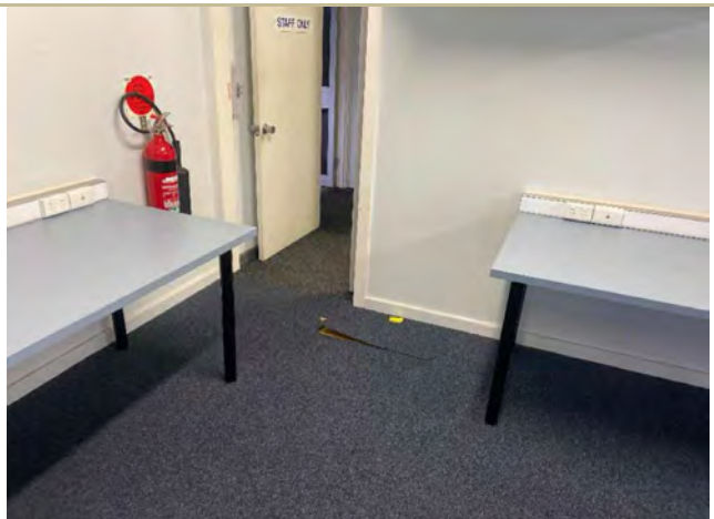
Item Number 2.1: Internal, L1, Beneath carpet, Northwest adjacent staff passage way, light blue tile, Vinyl Floor Tile and glue - Chrysotile
