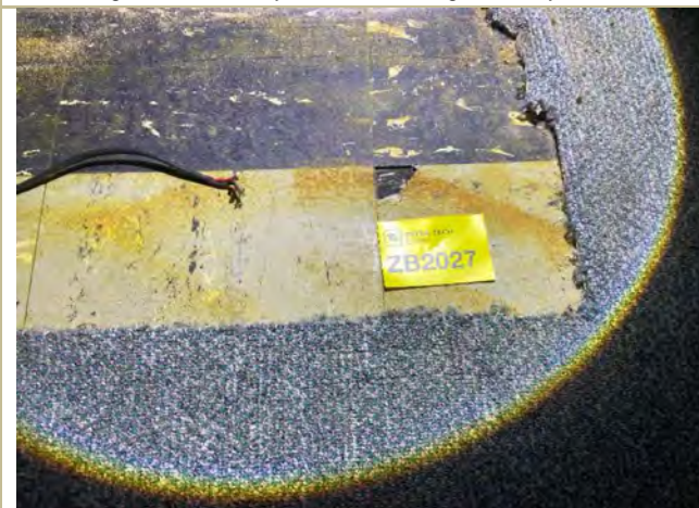
Item Number 5: Internal, L1, Beneath carpet cut out, south elevation, light grey tile and adhesive, Vinyl Floor Tile - Chrysotile
