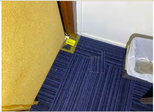
Item Number 1.1: Internal, L1, Beneath Carpet, west side, Vinyl Floor Tile and glue - Chrysotile
