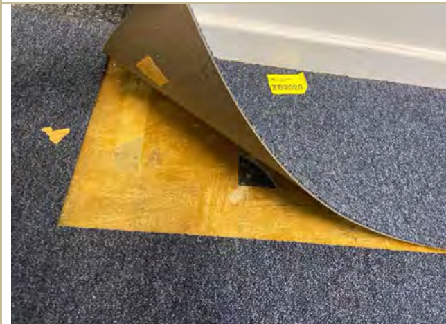
Item Number 2: Internal, L1, Beneath carpet, Northwest adjacent staff passage way, light blue tile, Vinyl Floor Tile and glue - Chrysotile
