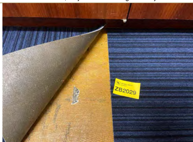
Item Number 8: Internal, L1, Admin office, central, beneath carpet, grey tile, Vinyl Floor Tile and adhesive - Chrysotile
