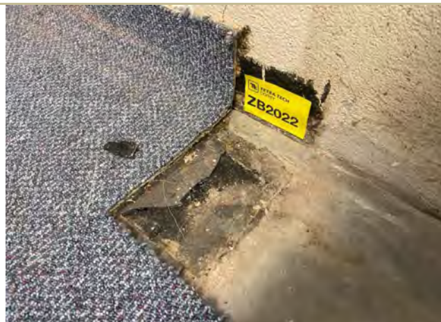
Item Number 7: Internal, L1, Beneath carpet, South East corner of room, Vinyl Floor Tile and glue - Chrysotile
